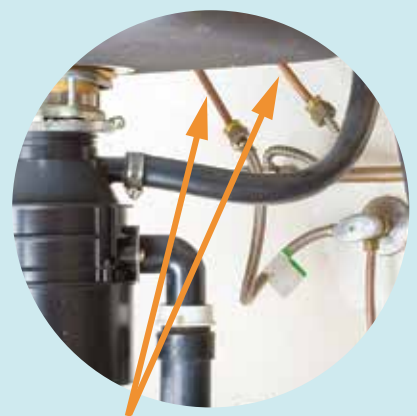
Do your water supply pipes look like a penny? Then they are copper!
