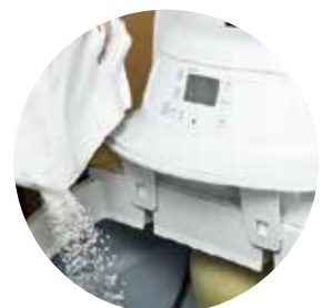
Water Softener (found inside or outside the house)
