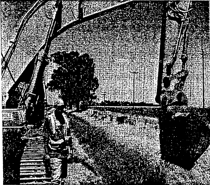
Excavator Operator Dennis Hennagin
